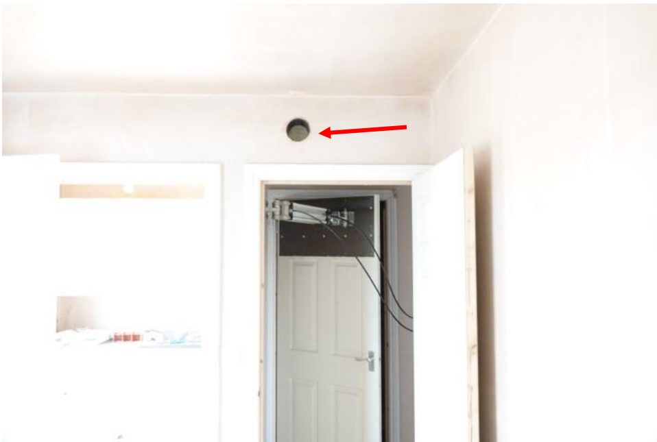
Figure 4: 100 mm diameter vent opening above kitchen door into hallway
