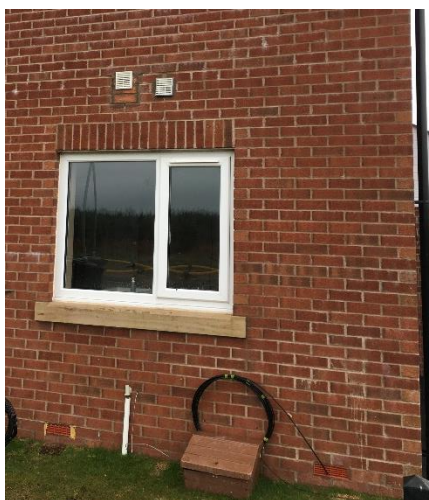
Figure 6: 78 cm 2 and 141 cm 2 ducted ceiling vents in kitchen
