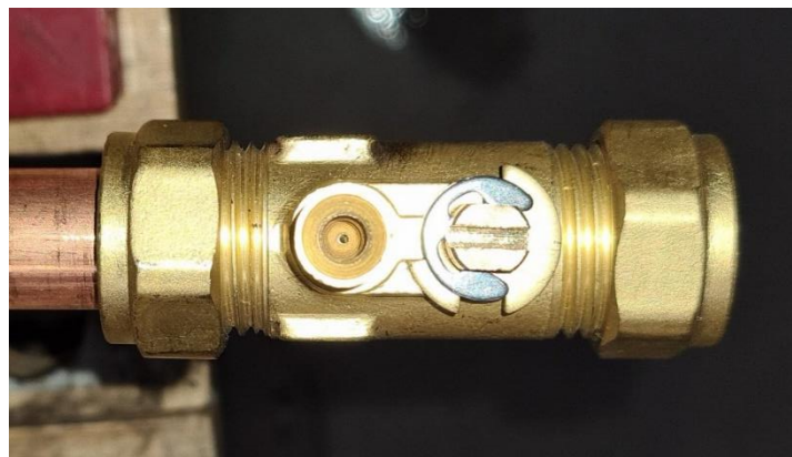
Figure 12: 1mmTP Purge point with detail of 1 mm purge hole
