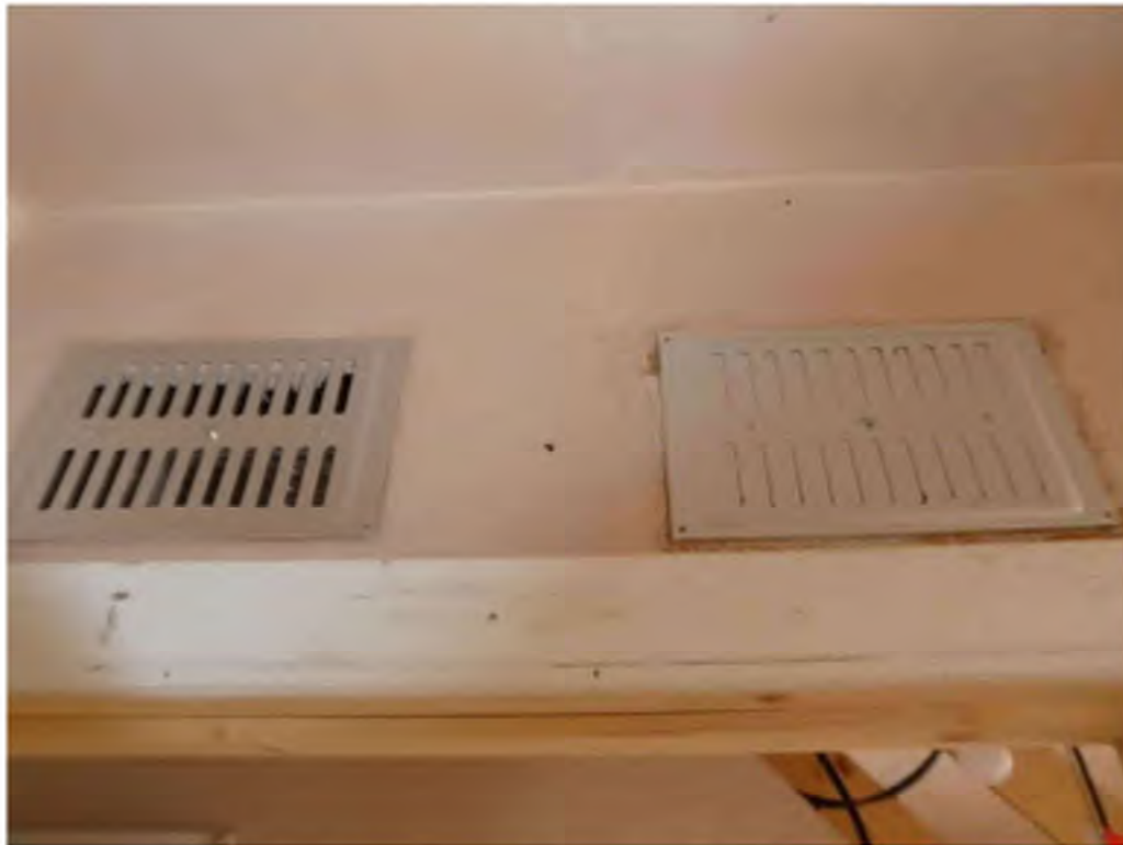
Figure 13: 85 cm 2 vents above living room door (one open, one closed)
