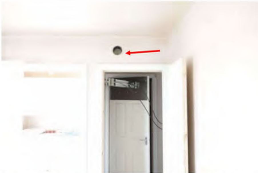
Figure 9: 100 mm diameter vent opening above kitchen door into hallway
