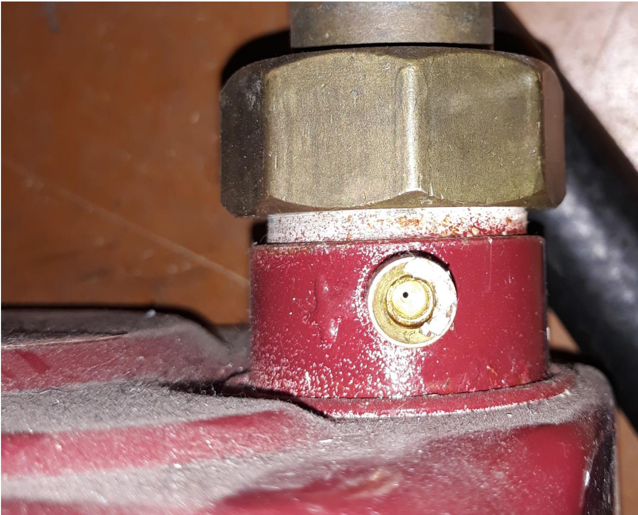
Figure 9: Meter test point, with small orifice visible
