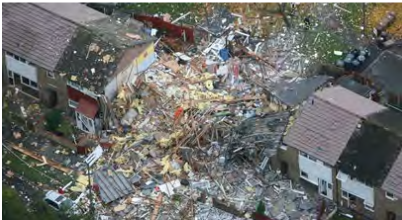
Figure 23: Damage to terraced housing following a domestic gas explosion in Salford – Greater Manchester in November 2010 (image from [21])
