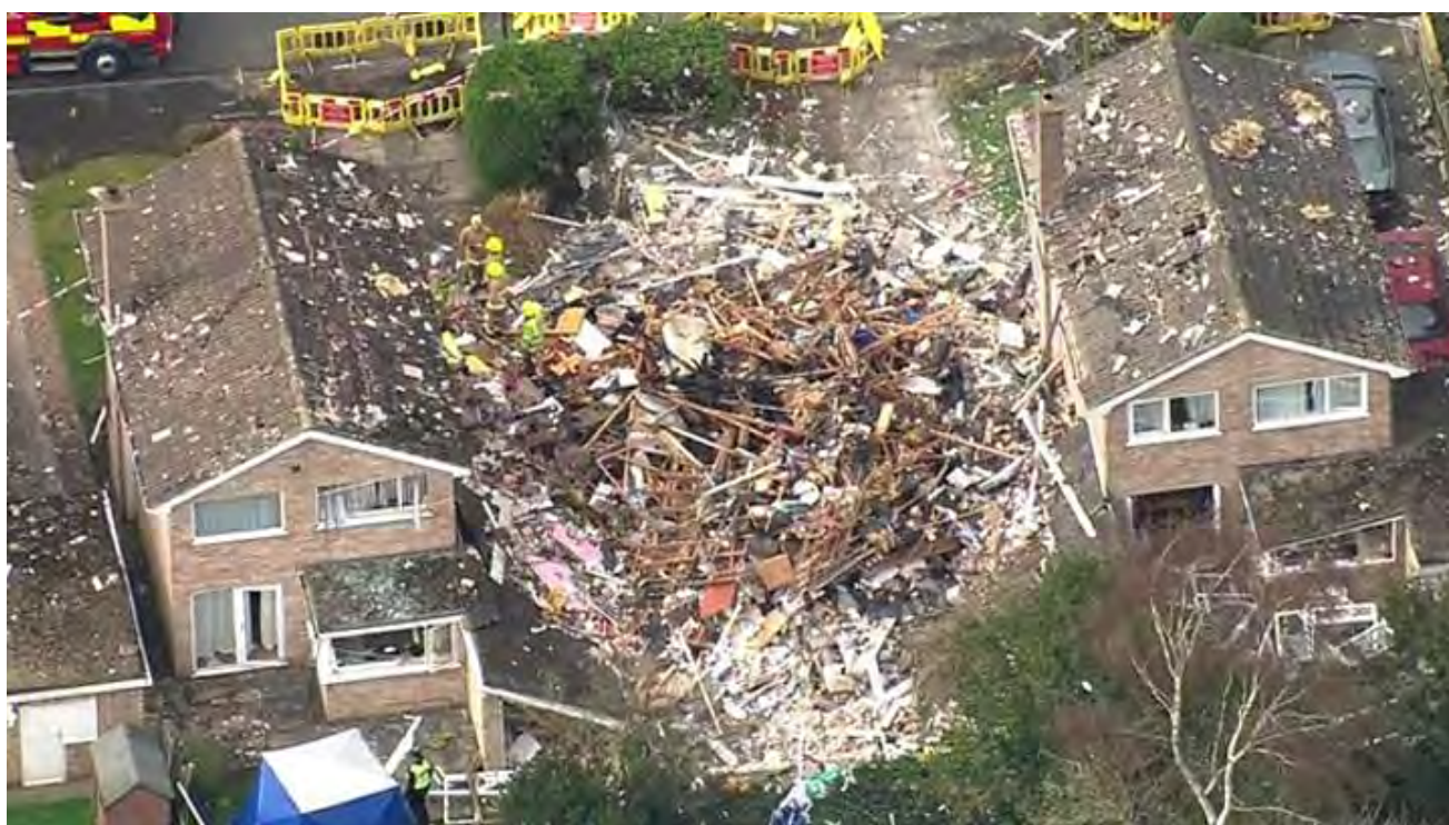
Figure 24: Damage to detached housing following a domestic gas explosion in Haxby – Yorkshire in February 2016 (image from [22])
