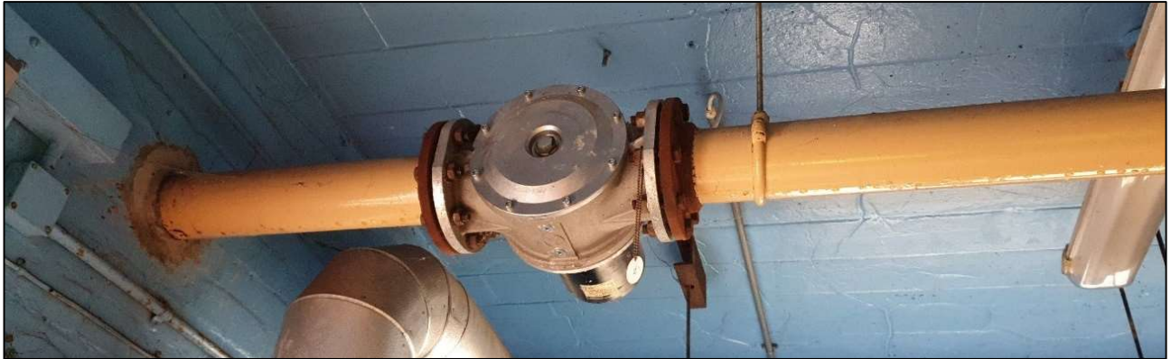
Figure 6: Electrically operated solenoid valve (SOV)
