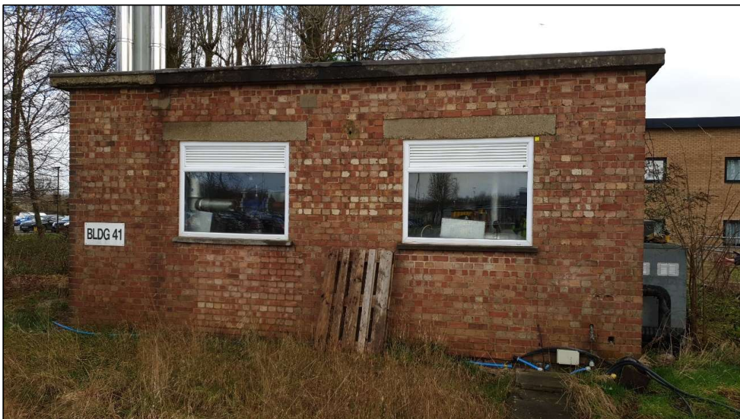
Figure 3: Looking east towards the plant room
