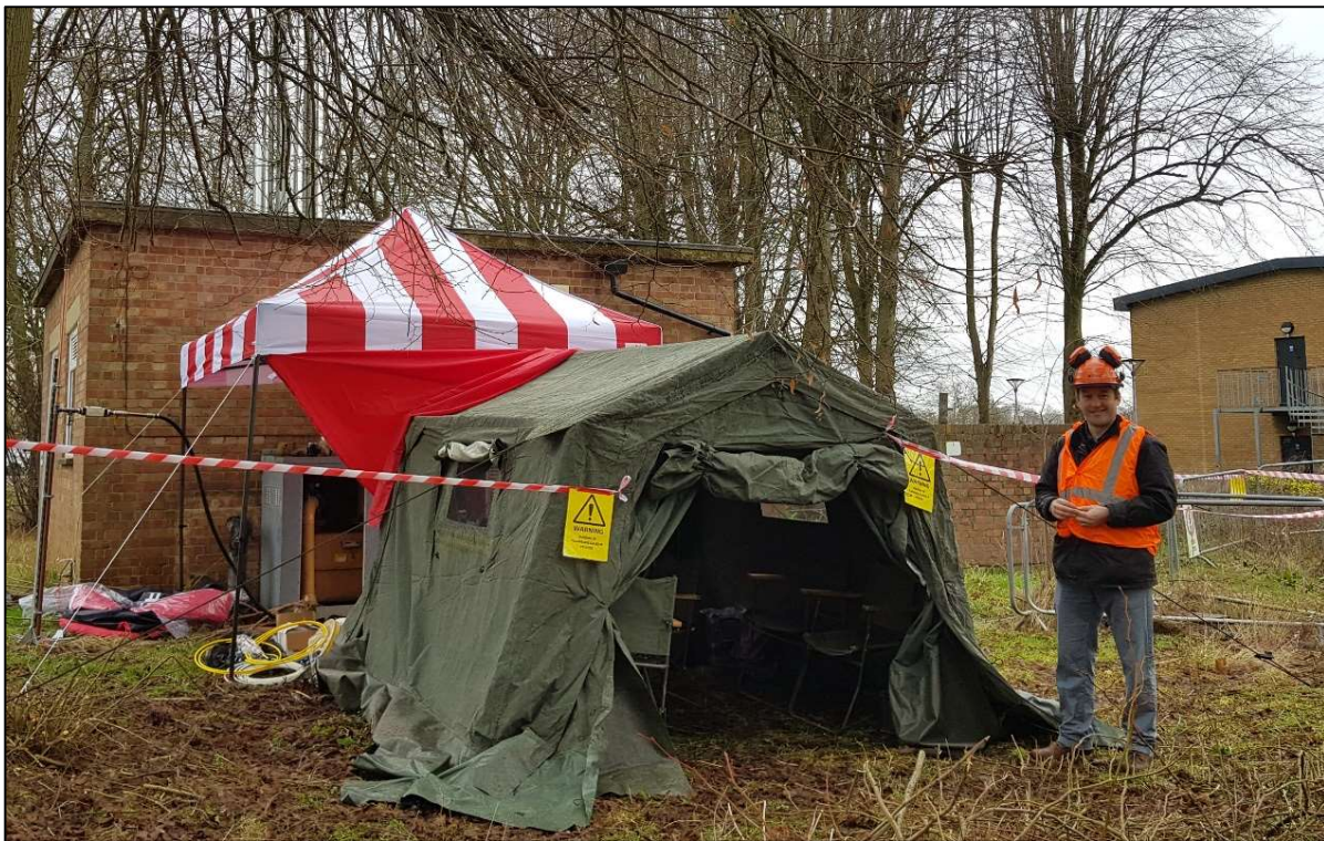
Figure 13: South side of the plant room with shelter and warning perimeter
