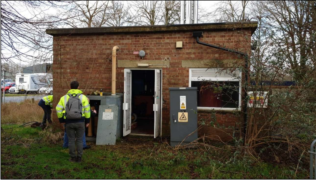
Figure 2: Looking north towards the plant room, building 41
