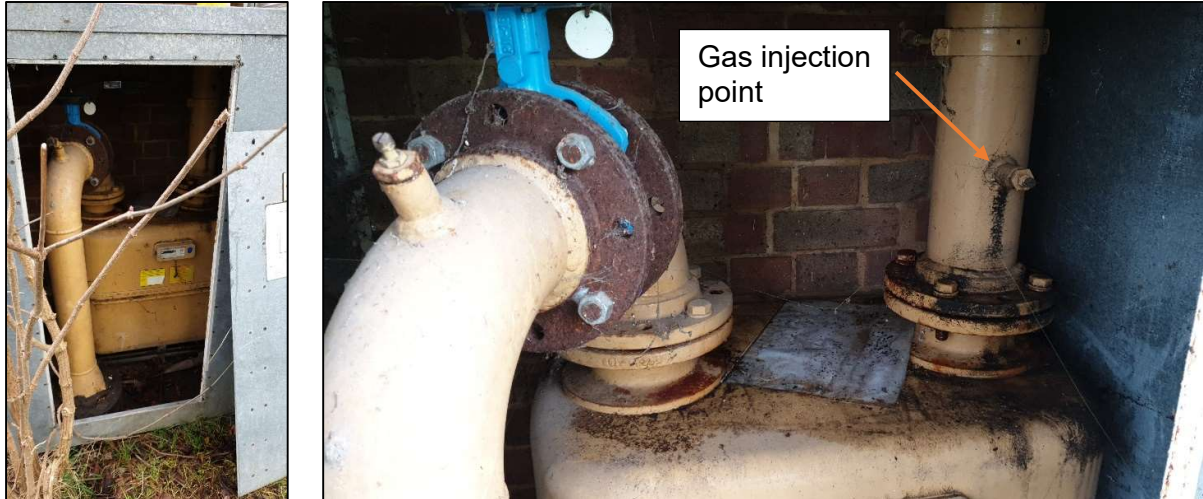
Figure 4: Meter cabinet with blue ECV and test point used for gas injection
