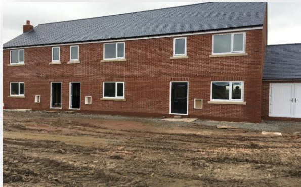
Mini housing complex, and 100mm pipeline network to distribute Hydrogen or methane
