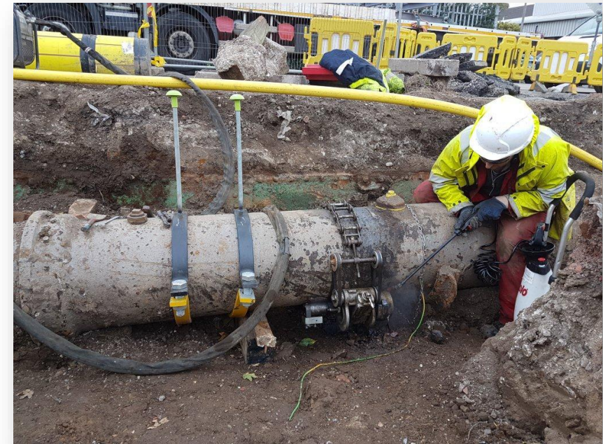
Large diameter iron test piece removal
